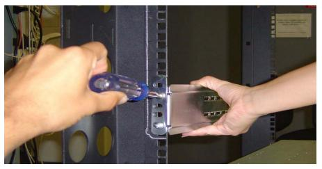
Figure 2-4: Attach Brackets to Post Separate from Shelf Unit
